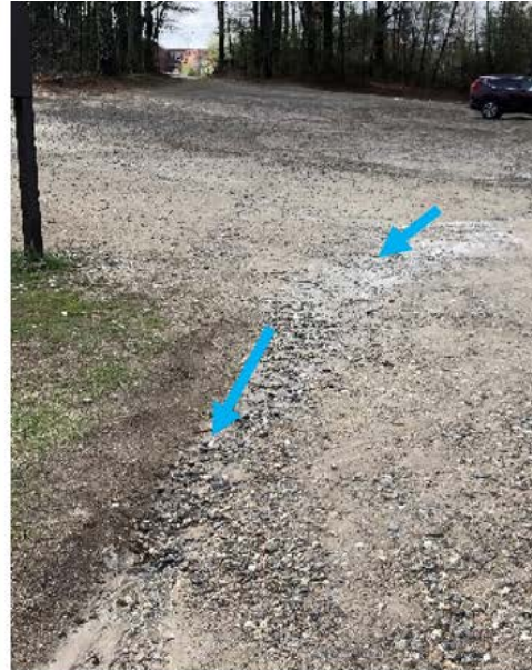
Photo 1-3: Dirt parking area eroding and washing into pond.
