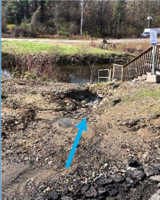
Photo 3-1: Severe erosion adjacent to water access point.
