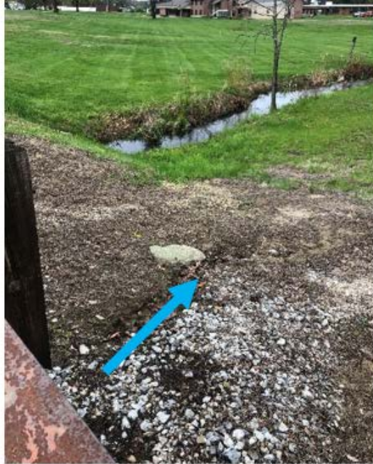
Photo 7-2: Edge of roadway erosion channel.
