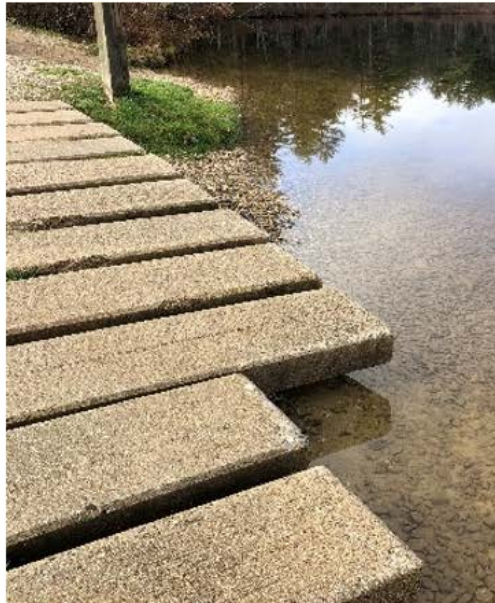
Photo 1-2: Concrete block boat ramp undercut.
